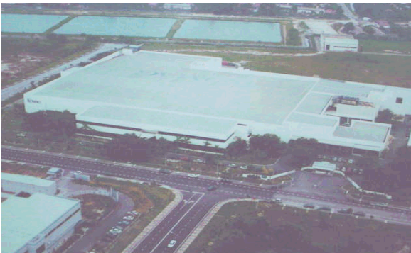
KOMAG Campus 3 Plant
