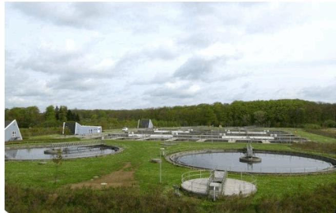
Removal of organic substance and nitrate occurs solely by biological principles. In 1999 the treatment plant was expanded with a biological sludge plant. Excess sludge from the wastewater treatment plant is treated here.
