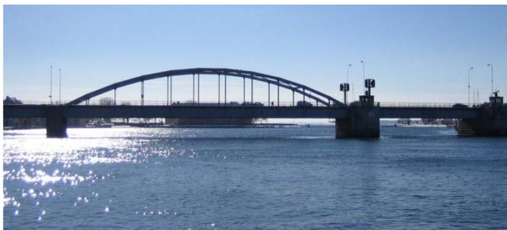
Before the modernization in 1996 and 1997, the motors used to operate the bridge flaps and sliding bolts were DC current injection engines. After the modernization, AC engines with frequency transformers were installed instead. At the same time, a new system for management, adjustment and surveillance of all the operations of the bridge was implemented.
